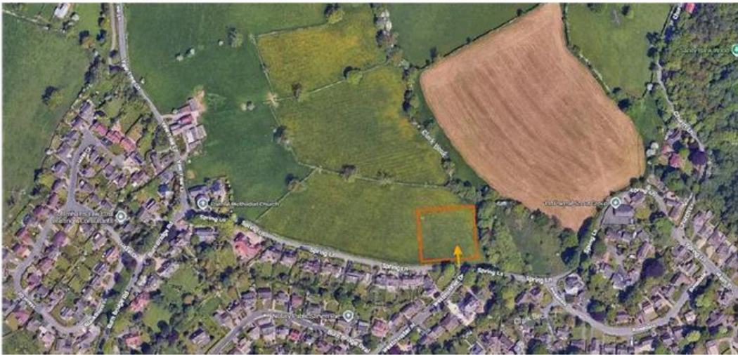
Spring Lane Sewage Pumping Station: Site Location and Entrance
